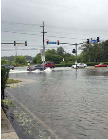
Front cover: Coastal flooding is of growing concern across Tidewater Virginia and in other coastal areas worldwide. Photo depicts flooding resulting from 2016 Hurricane Hermine in front of Norfolk's Larchmont Library at the intersection of Hampton Blvd. and Lexan Ave. on 9/3/2016 at 10:30 am EDT. Photo by J.D. Loftis/VIMS.
